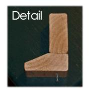
Nail-up the 2x4 and 2x2 (ten-penny spirals are great). Make awning tops of 2x2 and 1x4 (with a center support, as in illus.3), securing this frame to itself with screws, nails, and exterior glue. Roofing-nail the fiberglass to the wood. For these six windows two sheets of 26-inch by ten-foot fiberglass material were more than perfect.
