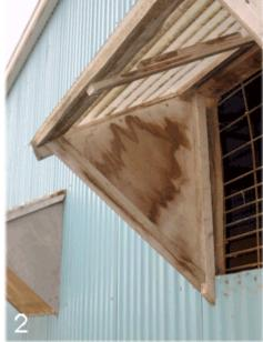
The idea is to get a shed-the-rain shape outside the building. Two-by-four trimmed so that there is a slanted, outside edge (to shed rain, to follow the awning's slant) is nailed-up to the underside of the barn's 2x4 structure (illus. "detail"). Two-by-two is
