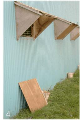
Seems to me I'd made cardboard templates for the 1/4 inch plywood sides (gussets), and remember that the top-point of both sides of each window gusset is trimmed-off squarely (for clearance, and do remember that the 2x2 covers any weather-leak (illus. 3). Caulk or use expanding foam to seal the top of the awning to the barn. I'd later trimmed strips of wood and fastened them just in from the lower edges of these gussets (illus. 2, 4).
